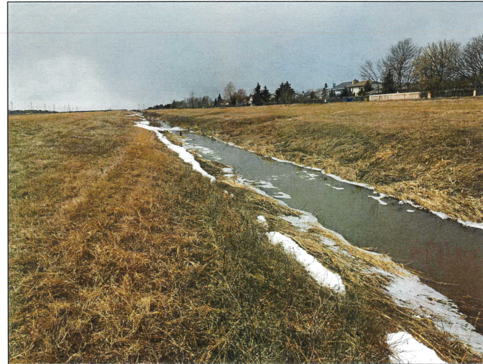
PHOTOGRAPH 7: FACING SOUTH WEST SHOWING THE LOT 16 DRAIN
